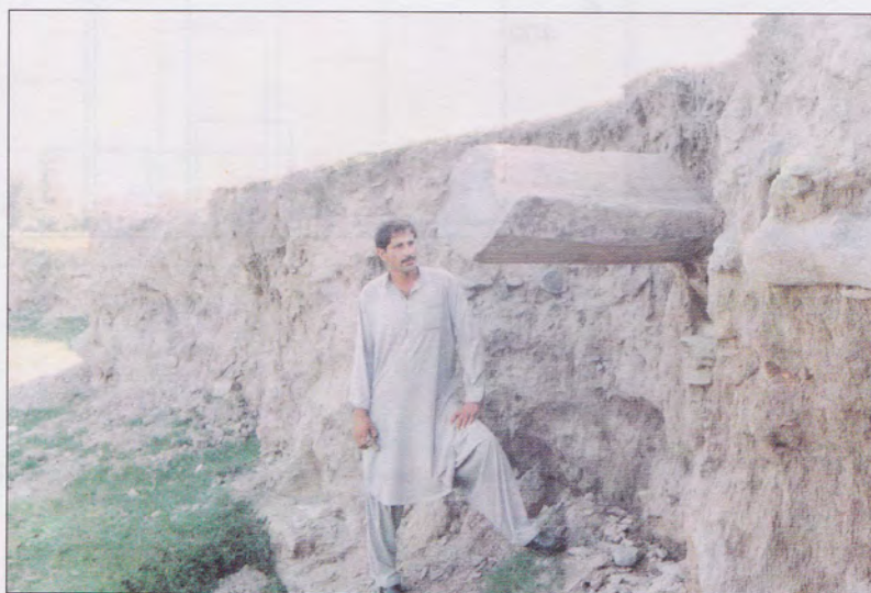
22. Megaliths used in the Kushan buildings at site no. 580
